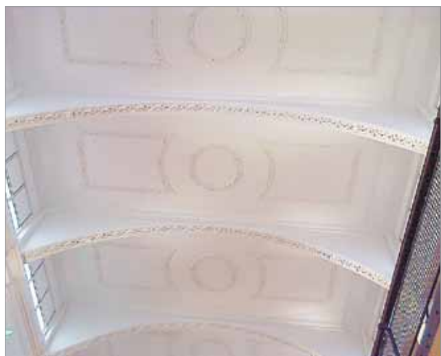
Detailed designed ceiling in the foyer of the Grand Pacific Hotel. Picture: JESSIE NAUA
