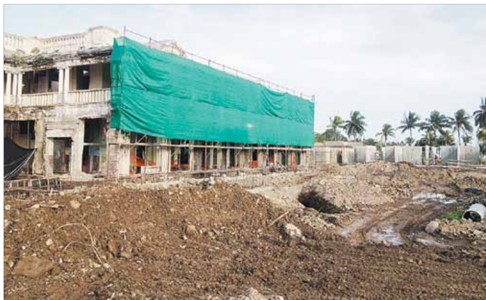
The Grand Pacific Hotel during renovations over the past two and a half years.
